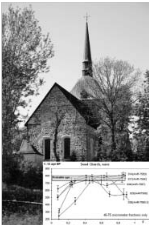
Figure 10. The church of Sund, Åland. Five profiles from the nave of the church suggest a building date at the second half of the 13 th Century, Aarhus. Photo Åsa Ringbom.
